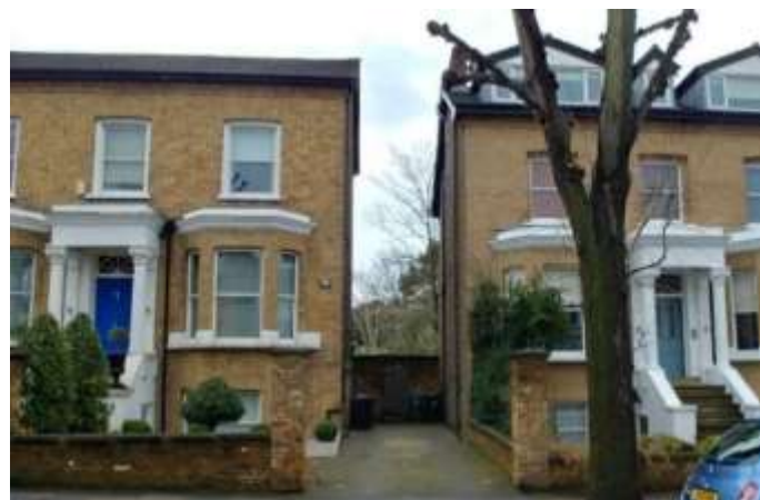
59 (and 57) Eaton Rise elevation – before
