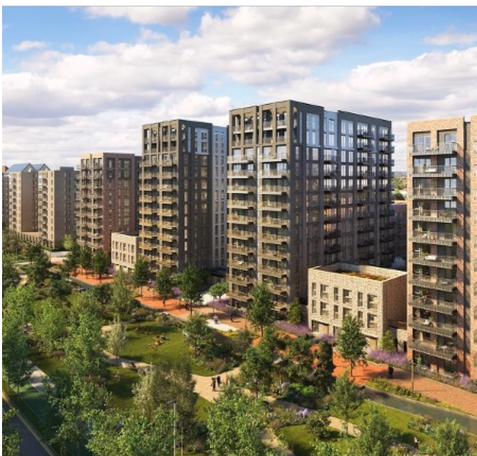
Berkeley Homes Gas Works (Green Quarter) scheme
